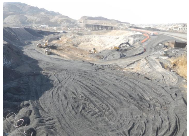
Slag excavation activities within the PBA Interim Channel
