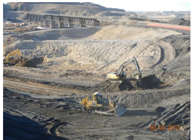
Slag excavation activities within the PBA Interim Channel
