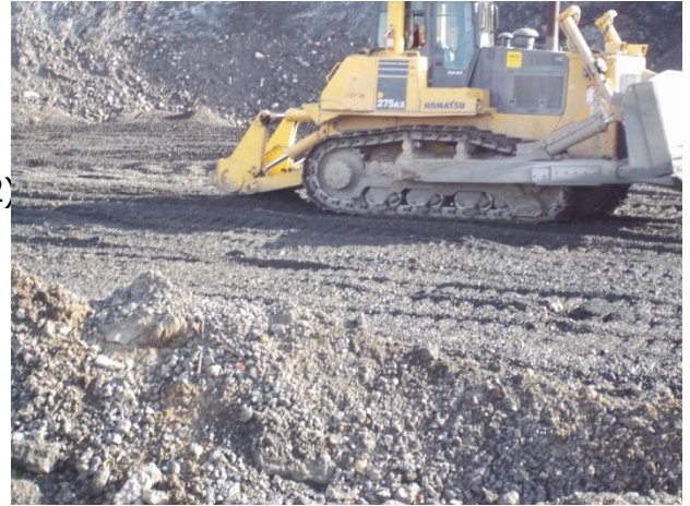
Ripping slag with a bulldozer equipped with a single tooth ripper within the PBA Interim Channel.
