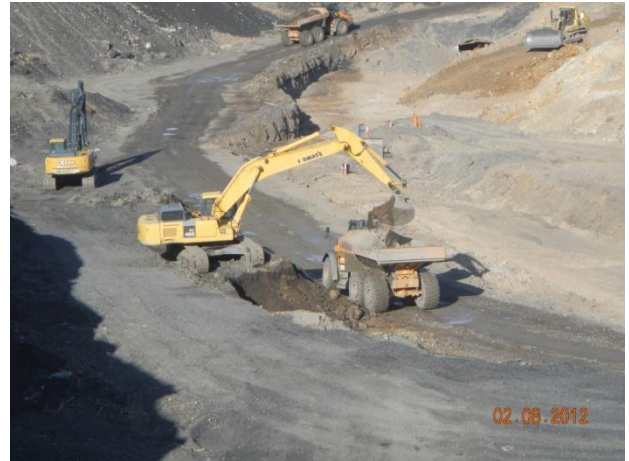
Loading targeted slag materials from within the PBA Interim Channel
