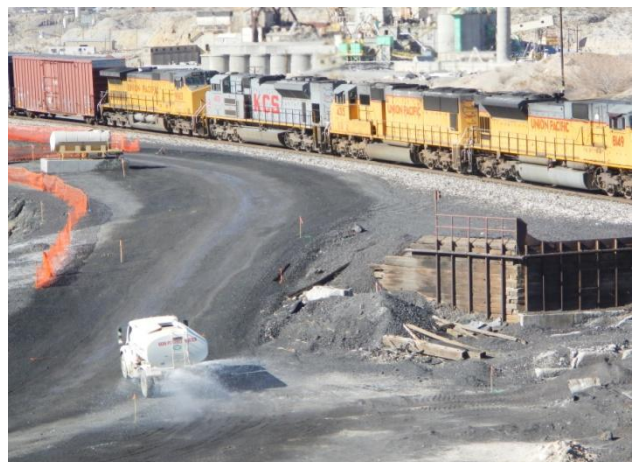
Applying water to temporary haul routes using a 2,000 gallon water truck.
