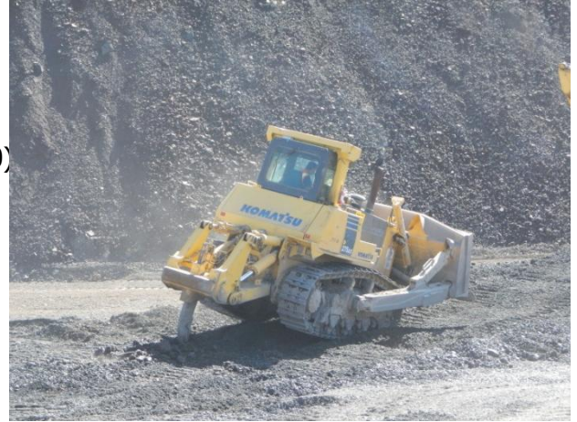
Ripping of slag material within the PBA Interim Channel.
