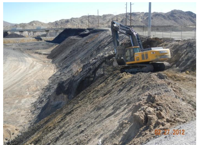
Bank stabilization activities located on adjacent PBA Interim Channel banks
