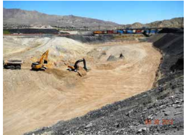
Excavation activities within the PBA Interim Channel
