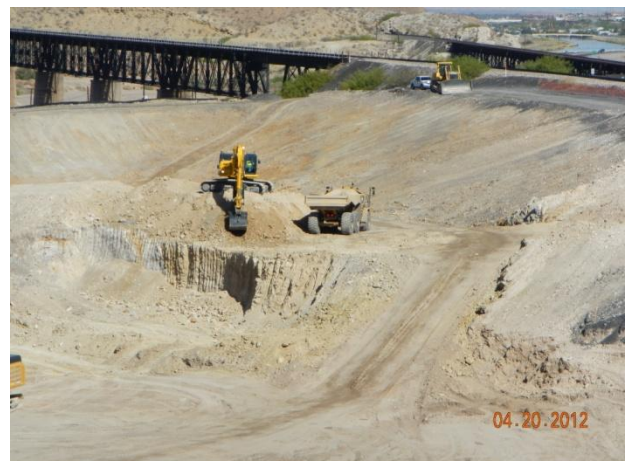
Excavation activities within the Category 1 Landfill footprint
