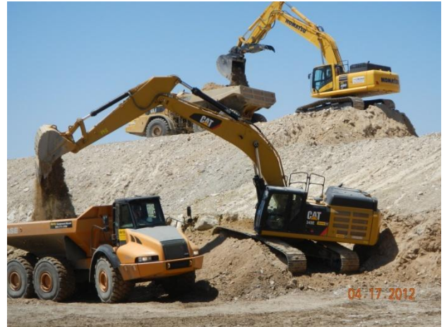
Excavation activities within the Category 1 Landfill footprint
