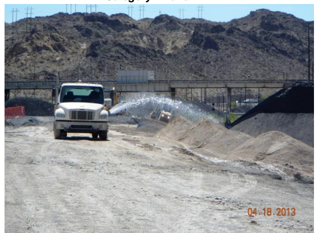
Installation of 6-inch prepared subgrade layer within Category 1 Landfill
