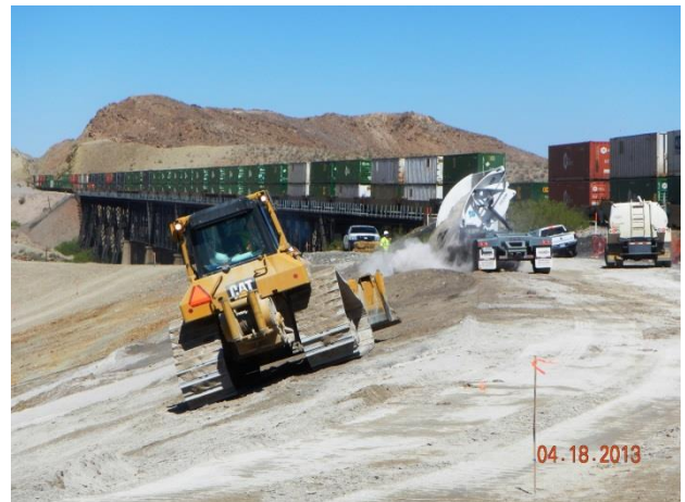
Installation of 6-inch prepared subgrade layer within Category 1 Landfill
