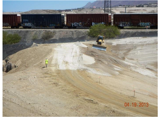
Grading of 6-inch prepared subgrade layer within Category 1 Landfill
