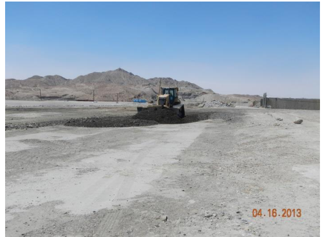
Placement of Category II material within the SW Fill Area.
