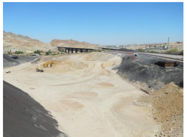
Excavation activities within the Category 1 Landfill footprint
