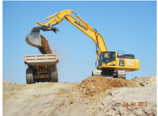
Excavation activities within the Category 1 Landfill footprint
