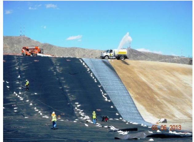
Geosynthetic installation activities within the Category 1 Landfill
