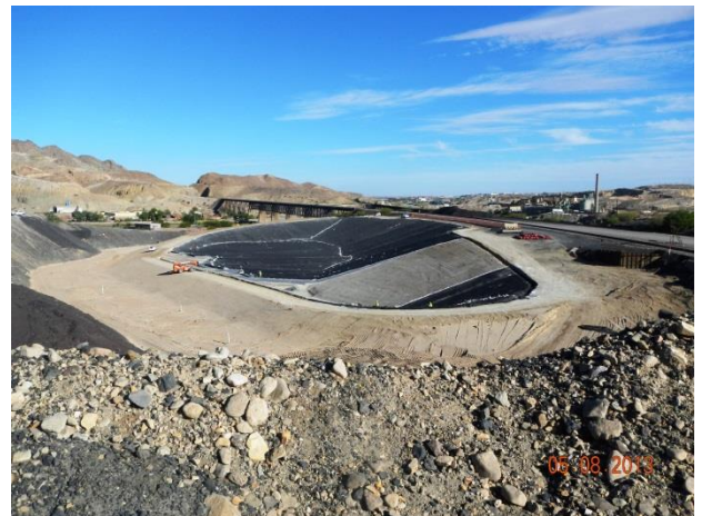
Current conditions within the Category 1 Landfill
