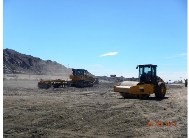
Mixing of crushed concrete with 12-inch minus material within the SW Fill Area using a hydraulic disc
