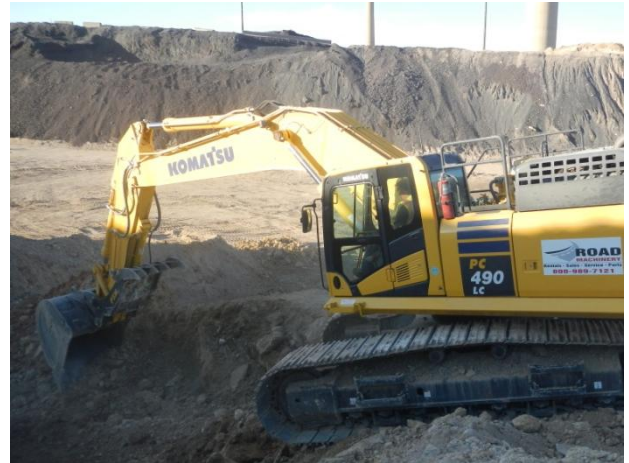
Excavation activities within the Category 1 Landfill footprint
