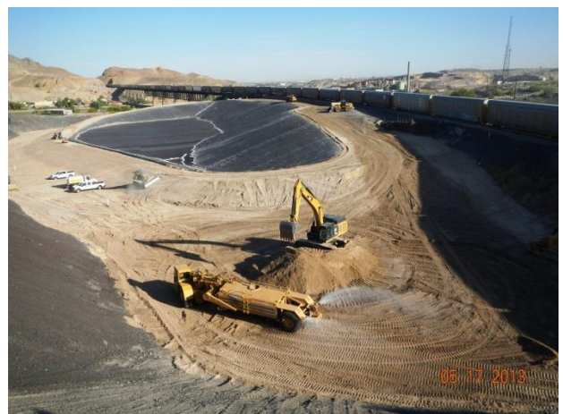
Grading activities within the PBA Channel
