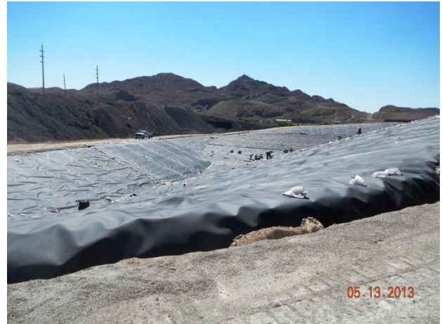
Geosynthetic installation activities within the Category 1 Landfill
