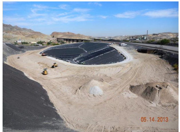
Current conditions within the Category 1 Landfill
