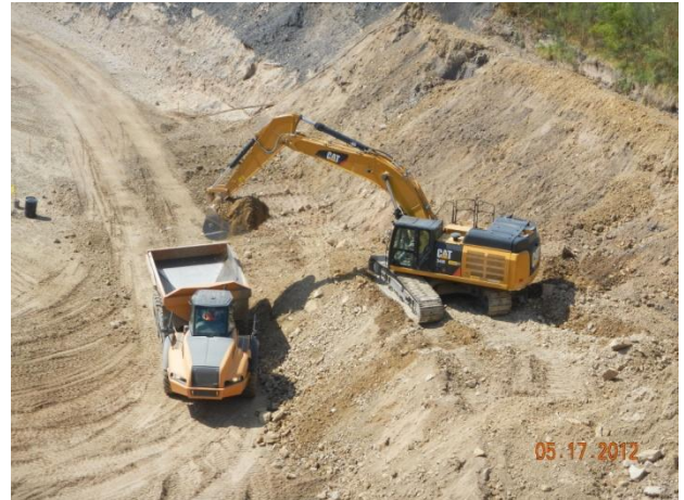
Excavation activities within the Category 1 Landfill footprint
