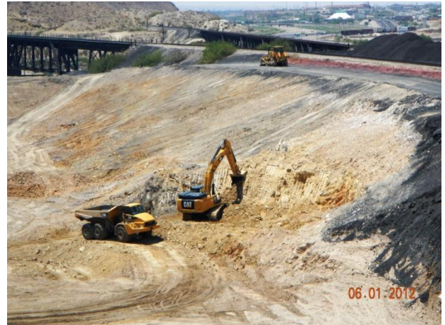
Excavation activities within the Category 1 Landfill footprint
