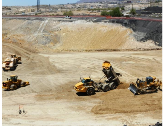
Structural backfill placement within the Category 1 Landfill footprint
