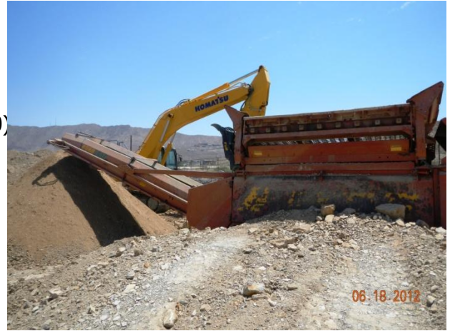
Screening and loading structural backfill materials.
