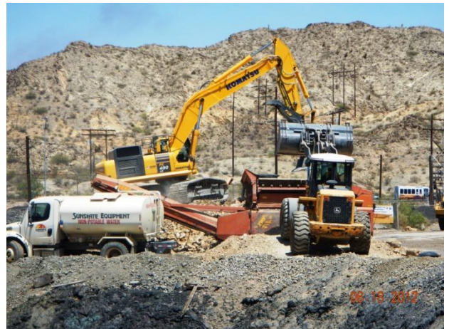
Material processing activities associated with mobile screen
