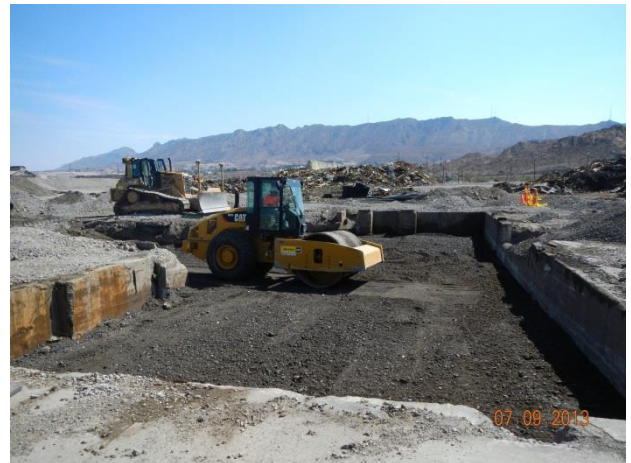
Backfill activities within a former plant basement
