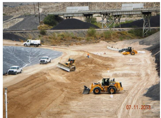
Subgrade preparation along PBA Channel slope
