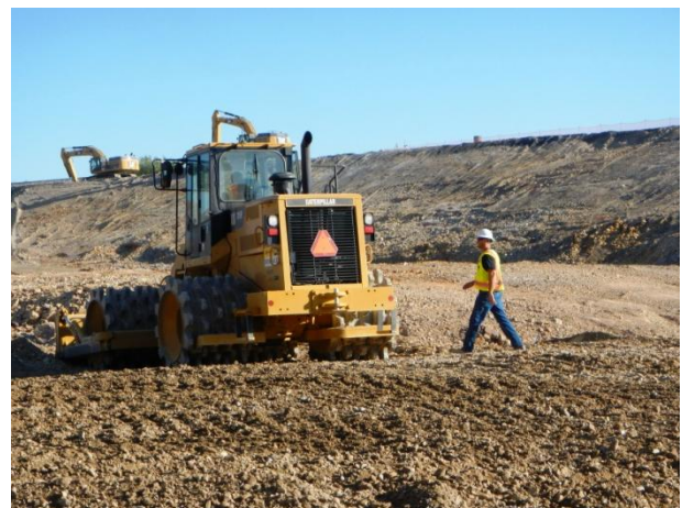
Compaction of structural fill using an 815 compactor
