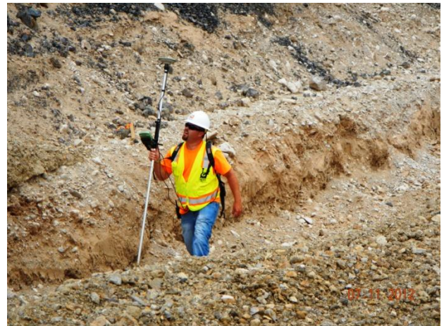
Interim construction survey using RTK GPS
