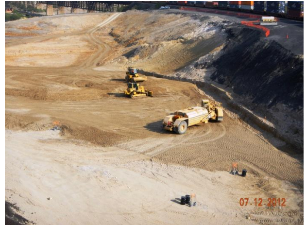
Structural backfill placement within the Category 1 Landfill footprint
