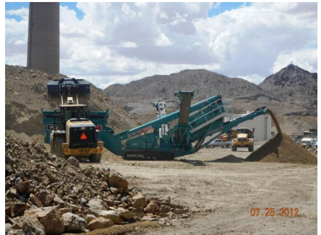
Material processing activities associated with mobile screen
