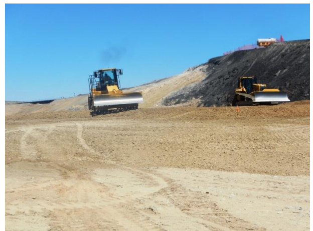
Grading and compacting structural fill
