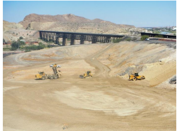
Structural backfill placement and compaction within the Category 1 Landfill footprint
