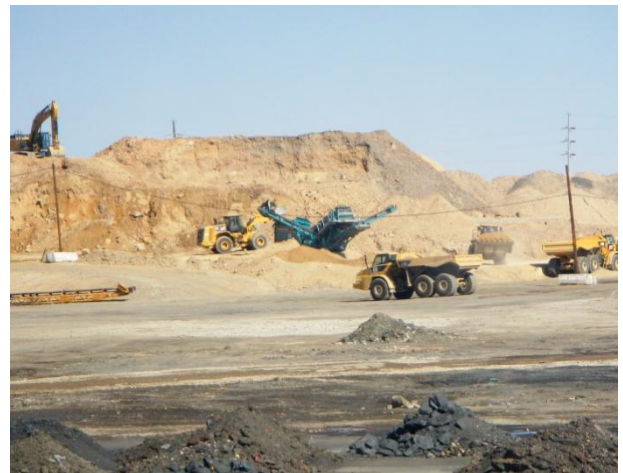
Material processing activities associated with mobile screen
