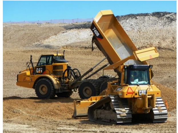
Structural backfill placement and grading
