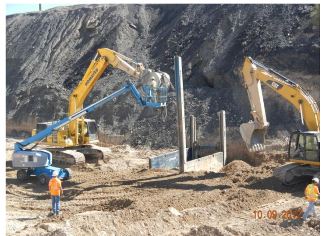
Removal of slide rail rigging using a hydraulic man-lift
