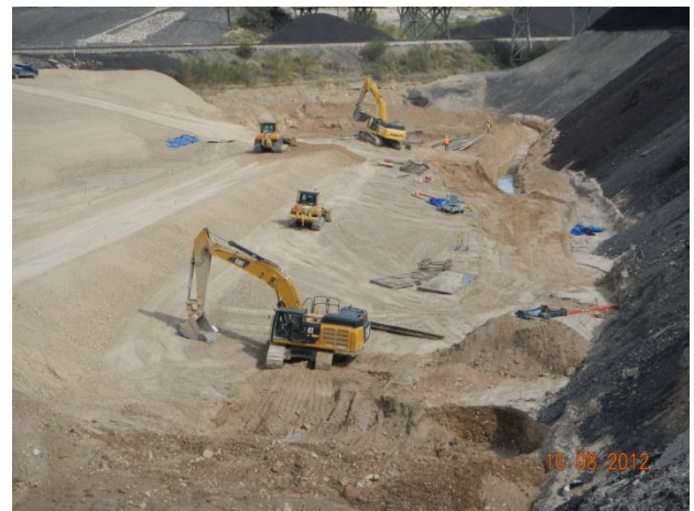
PBA and CAT 1 Landfill current conditions
