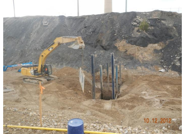
Installation of slide rail system components
