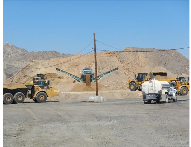
Screening existing stockpile soils to meet 3-inch minus specifications.
