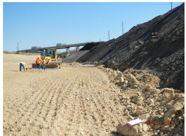
Conducting field nuclear density testing within compacted lift.
