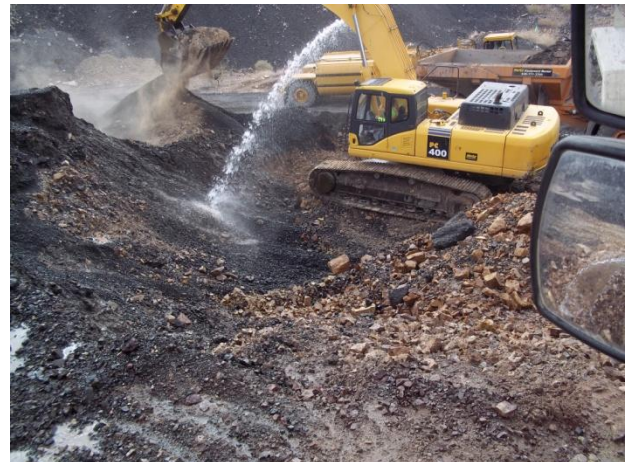
Slag excavation within the Category 1 Landfill footprint.
