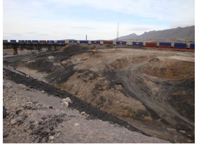
Excavation of Slag from Southwest corner of Category 1 Landfill.
