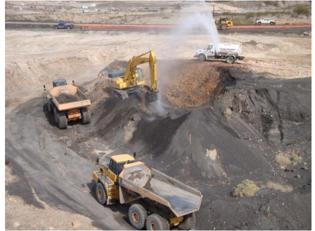
Loading Slag from within the Category 1 Landfill footprint.
