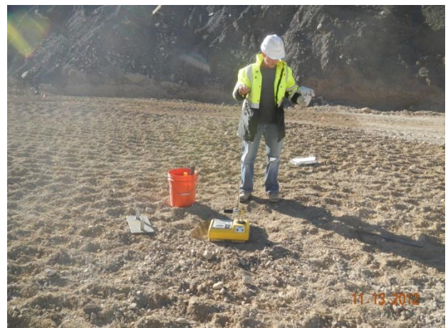
Performing field density testing on compacted backfill within the PBA channel.
