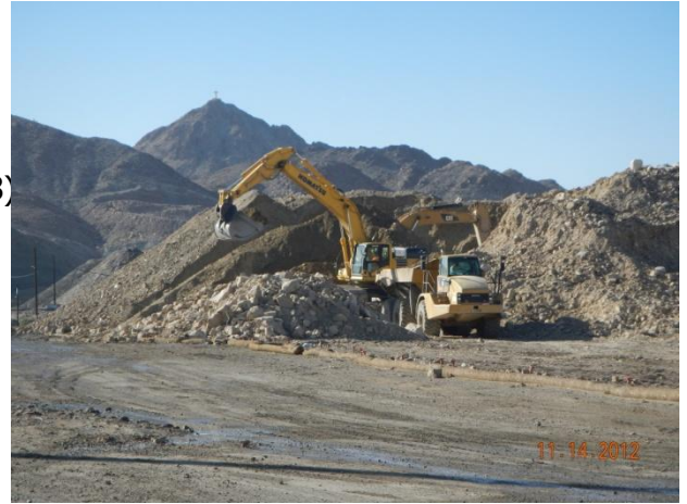
Loading of clean backfill materials
