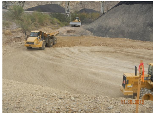
Installing loose lifts of backfill materials within PBA channel.
