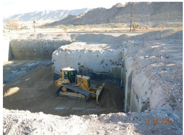
Placement of CAT II soils within the Ore Unloading Basement
