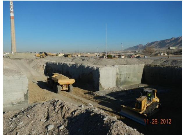
Installation of CAT II soils within the Ore Unloading Basement
