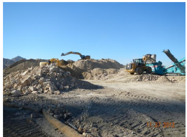
Screening of CAT II soils for Ore Unloading Basement
