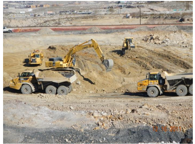
Loading targeted mass excavation materials from within the Category 1 Landfill footprint.
