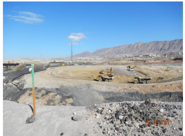
Excavation activities within the Category 1 Landfill footprint.
