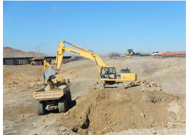
Loading targeted mass excavation materials from within the Category 1 Landfill footprint.
