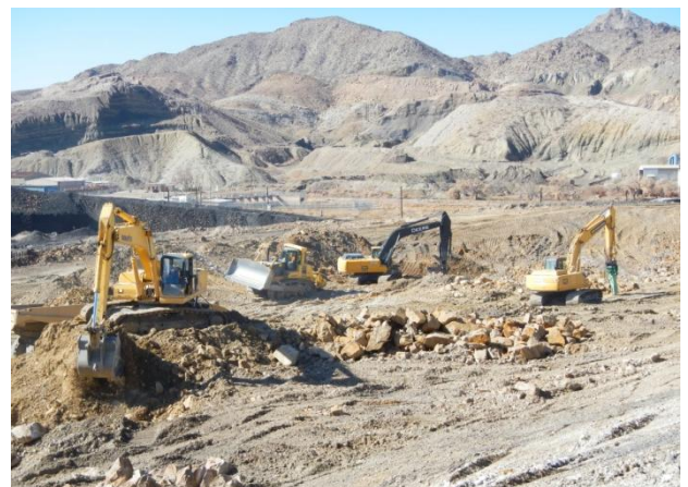
Excavation activities within the Category 1 Landfill footprint.
