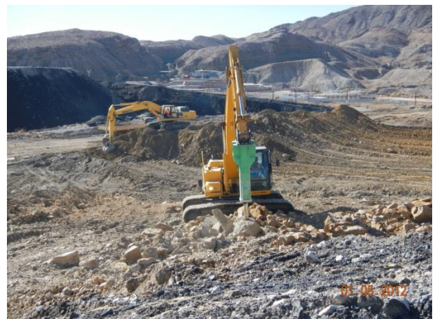
Breaking dense rock layer with a hydraulic breaker attached to an excavator.
