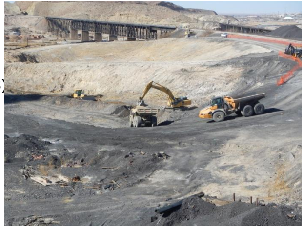
Slag excavation within the Category 1 Landfill footprint.
