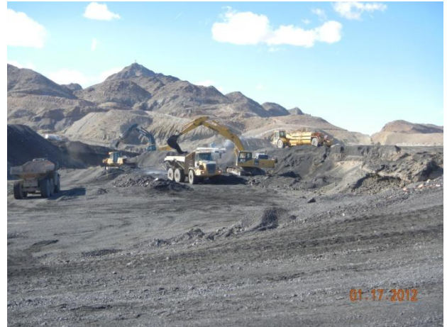
Loading targeted slag materials from within the Category 1 Landfill footprint.
