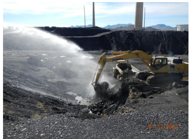
Slag excavation and dust suppression within the Category 1 Landfill footprint.
