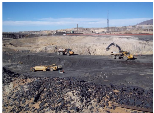
Slag excavation activities within the Category 1 Landfill footprint.
