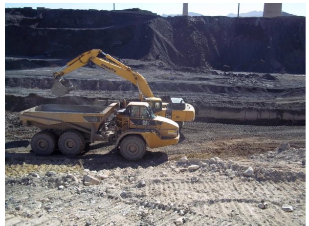
Sanitary/Storm sewer removal activities within the Category 1 Landfill footprint.
