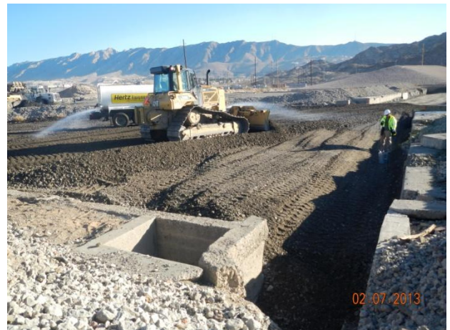
Grading of Category II backfill within the Engineering Trench
