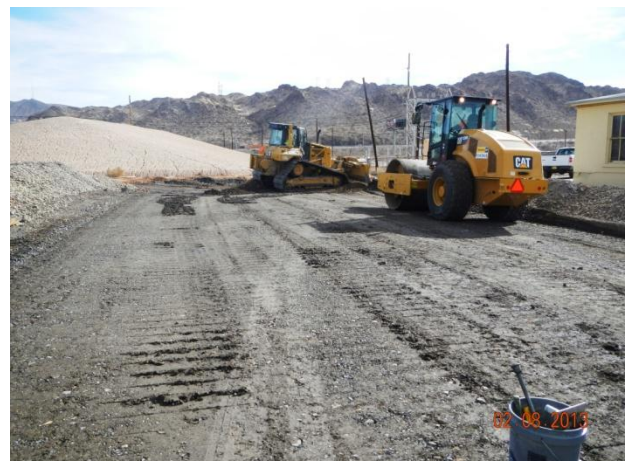
Category II soil compaction within the Engineering Trench
