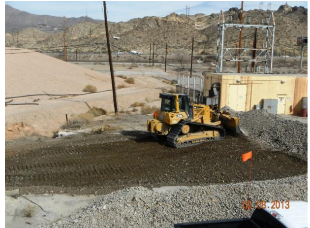
Grading of Category II backfill within the Engineering Trench
