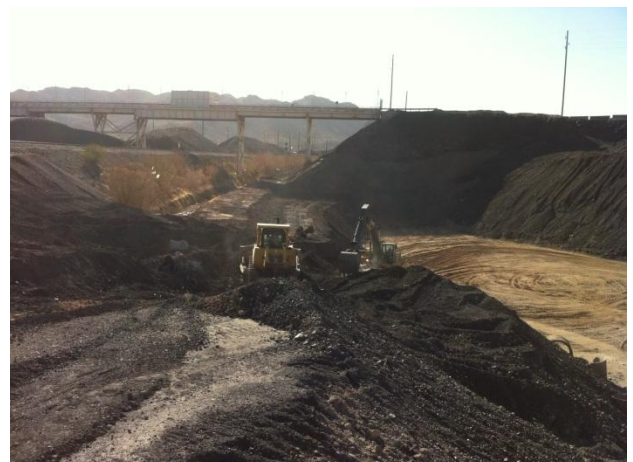
Excavation of slag material from within the PBA Interim Channel banks
