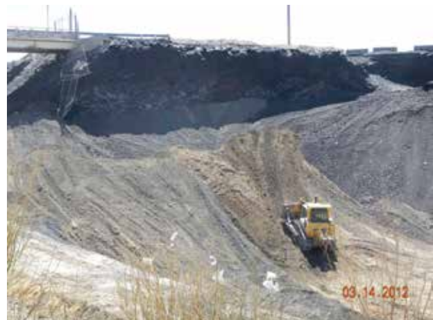
Construction of a temporary earthen buttress within the PBA Interim Channel
