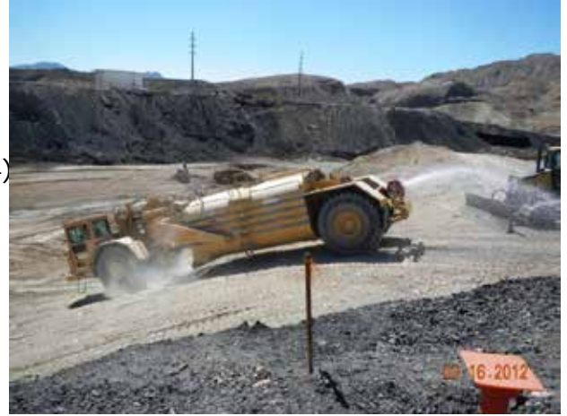
Applying water for fugitive dust control within the PBA Interim Channel
