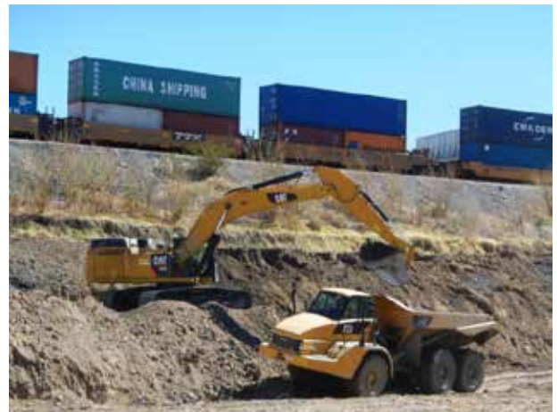
Loading of slag material within the PBA Interim Channel
