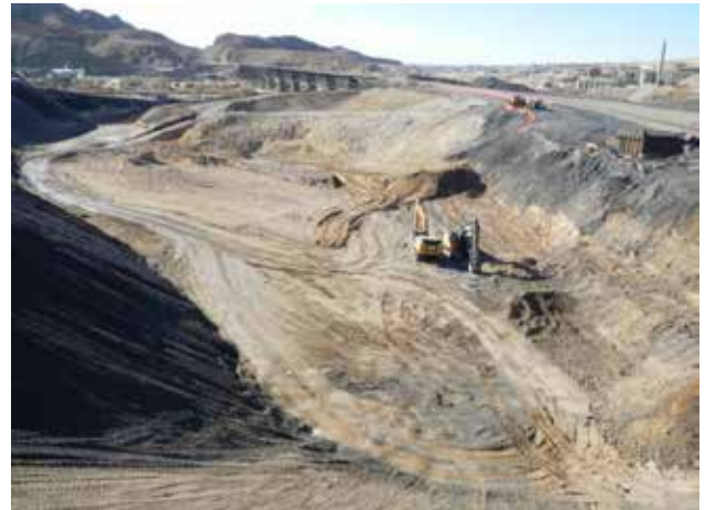
Excavation activities within the PBA Interim Channel
