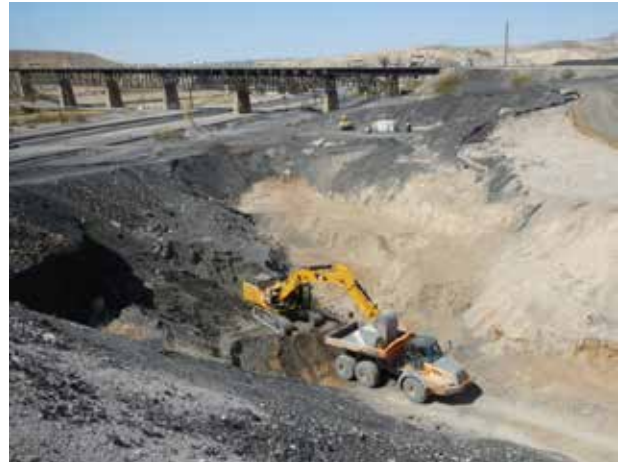
Excavation activities within the PBA Interim Channel
