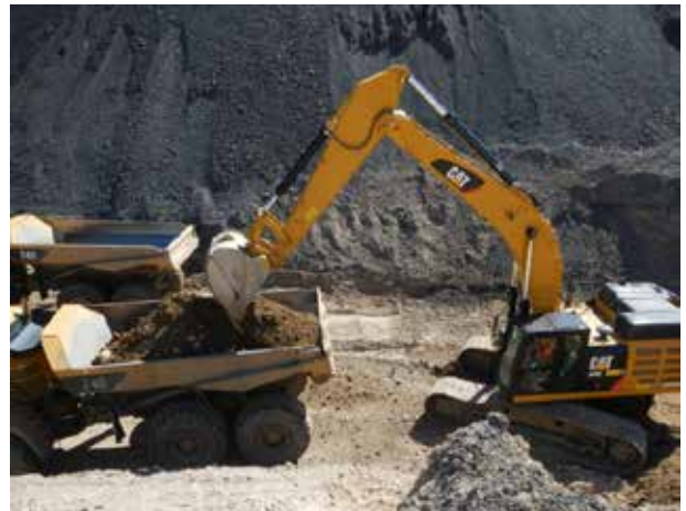
Loading of impacted soil beneath slag material within the PBA Interim Channel
