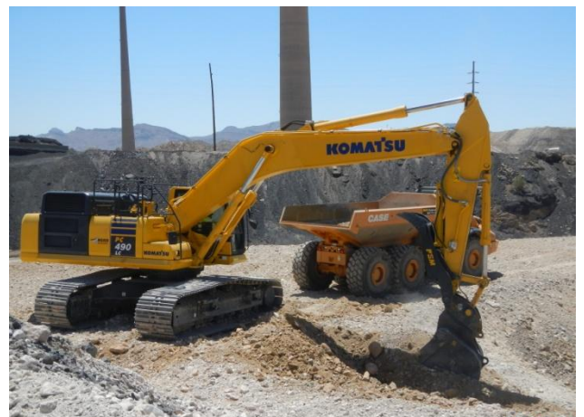
Excavation activities within the Category 1 Landfill footprint
