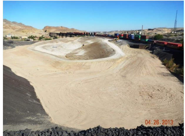
Current conditions of 6-inch prepared subgrade layer within Category 1 Landfill
