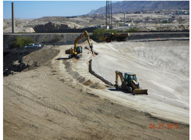
Excavation of the Category I Landfill geosynthetic anchor trench
