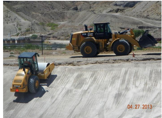
Compaction of 6-inch prepared subgrade layer within Category 1 Landfill
