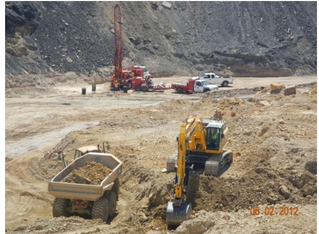
Excavation activities within the Category 1 Landfill footprint
