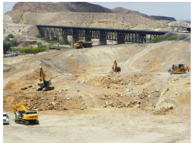
Excavation, loading and grading activities within the Category 1 Landfill footprint
