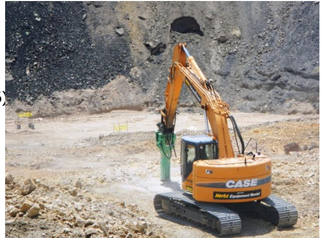
Hydraulic Breaker activities within the Category 1 Landfill footprint
