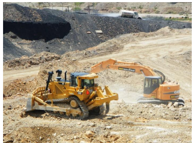
Excavation and ripping activities within the Category 1 Landfill footprint
