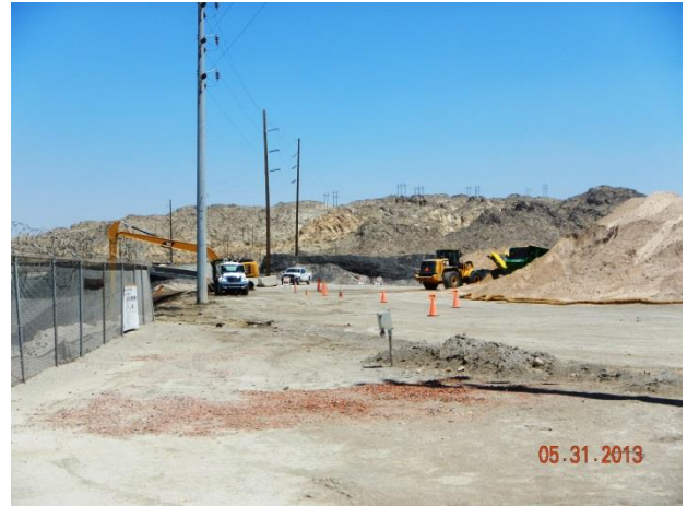
Site setup associated with the plant slope
