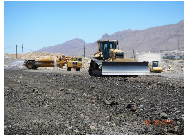
Grading, moisture conditioning and compacting Category II materials
