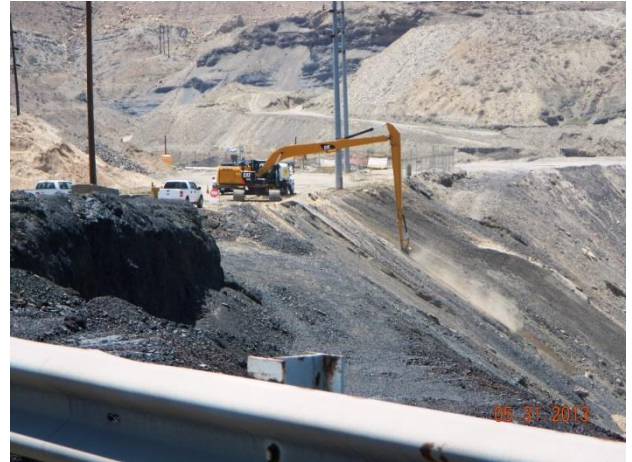
Plant slope stabilization activities within Area 2.
