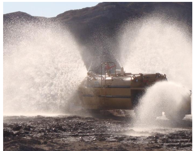
Dust suppression activities using a 10,000 gallon water pull.
