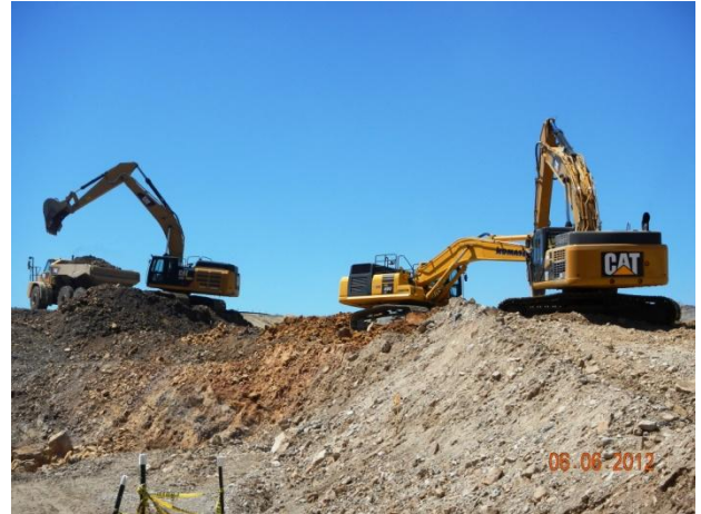
Excavation activities within the Category 1 Landfill footprint
