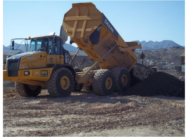
Stockpiling excavated slag materials.
