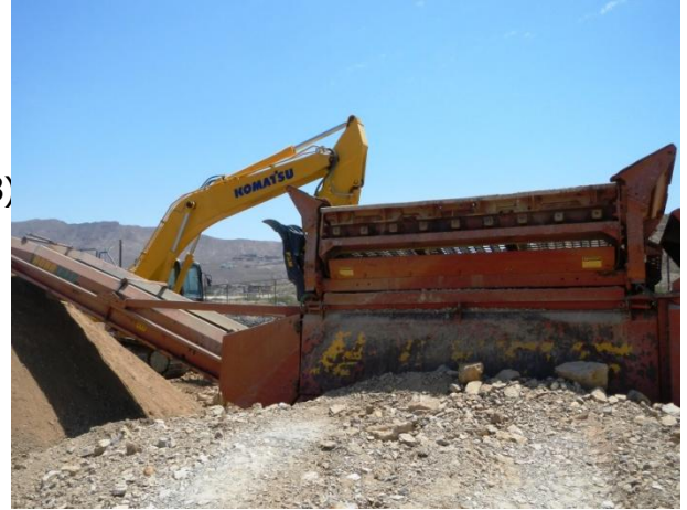
Stockpiling excavated slag materials.
