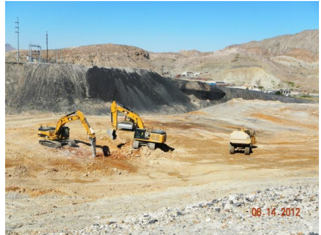
Excavation activities within the Category 1 Landfill footprint
