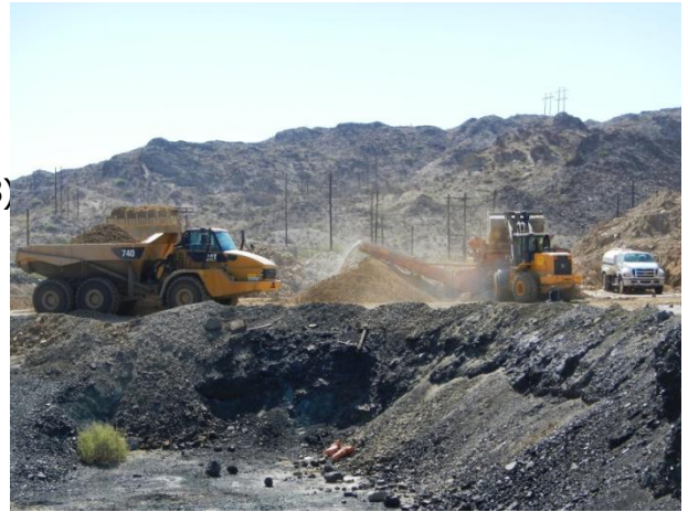
Screening and loading structural backfill materials.
