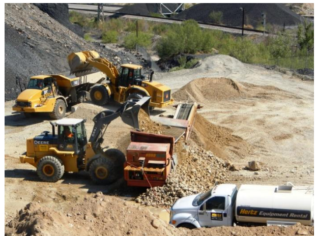
Material processing activities associated with mobile screen
