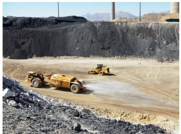
Moisture conditioning and compaction associated with structural backfill materials.
