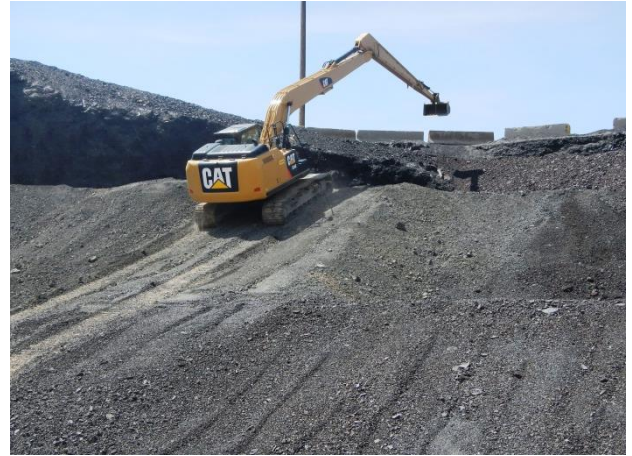
Plant slope stabilization activities within Area 3
