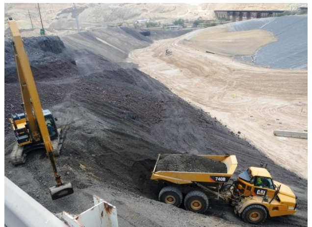
Plant slope stabilization activities within Area 3
