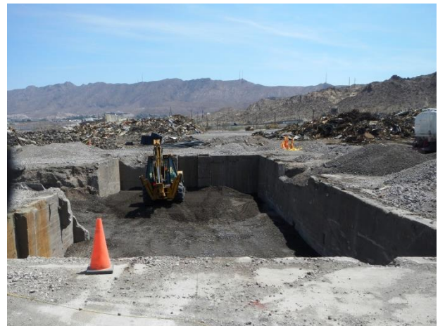
Backfill activities within a former plant basement
