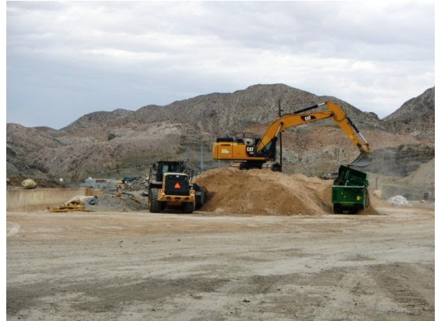
Screening select protective layer materials to be placed within the CAT 1 Landfill
