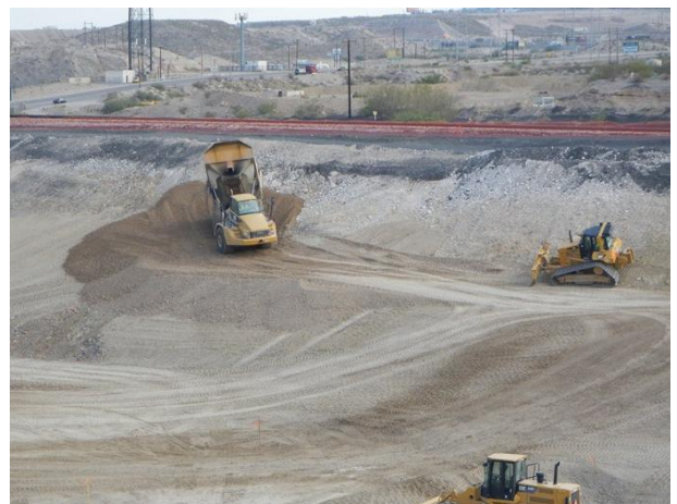
Grading and compacting structural fill
