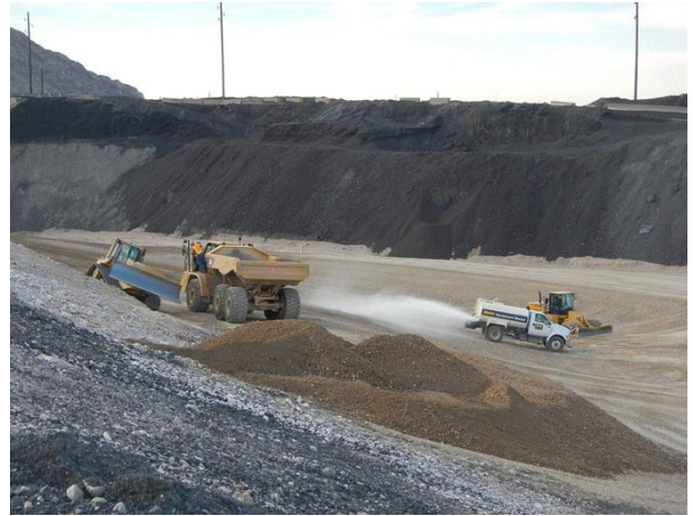
Placing, grading and moisture conditioning of structural fill
