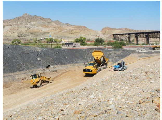
Structural backfill placement and compaction
