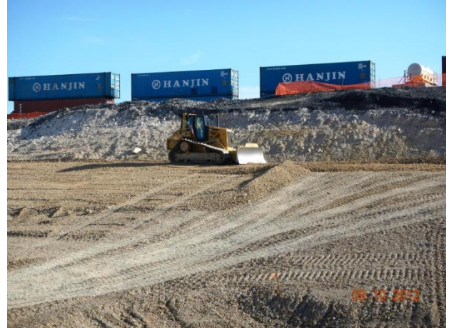
Grading of structural fill along CAT 1 Landfill slopes
