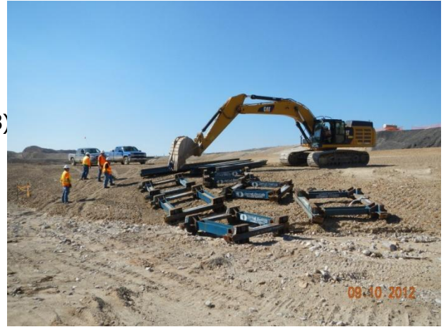
Assembly of slide rail components for PRB 1
