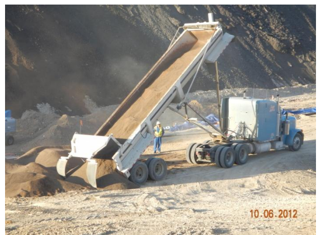
Delivery of ZVI backfill near PRB 1 location
