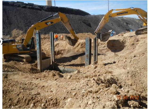
Installation of ZVI backfill within PRB 1
