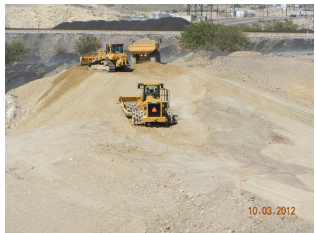
Backfill activities within CAT 1 Landfill footprint
