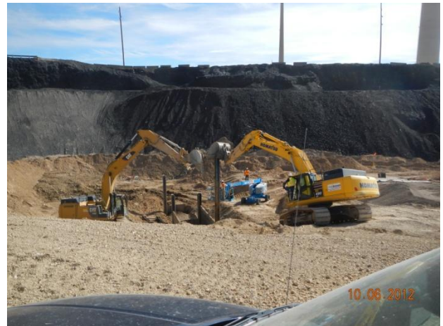
Installation of slide rail system components
