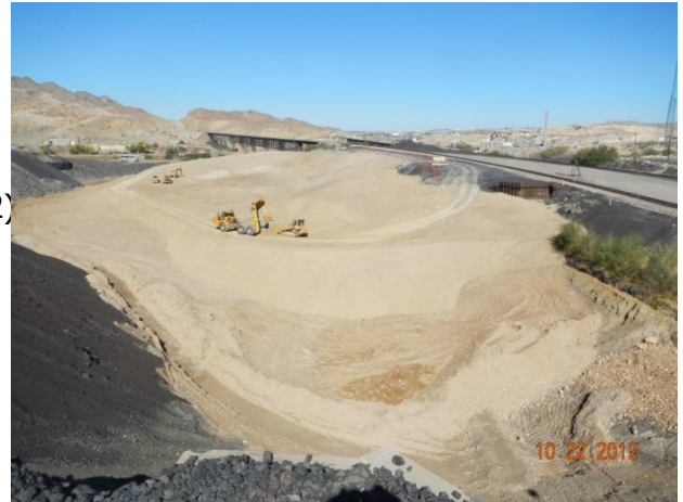
Installation of structural fill materials within CAT 1 Landfill footprint.
