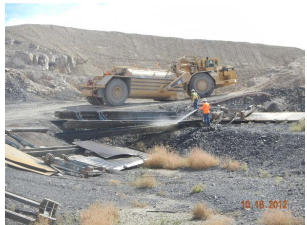
Demobilization of slide rail system associated with PRBs.
