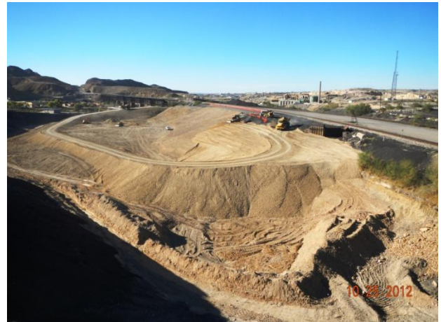
PBA and CAT 1 Landfill current conditions
