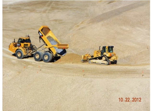
Installation of structural fill within CAT 1 Landfill footprint.
