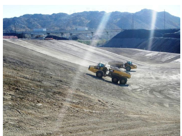
Hauling of backfill materials using articulated dump trucks
