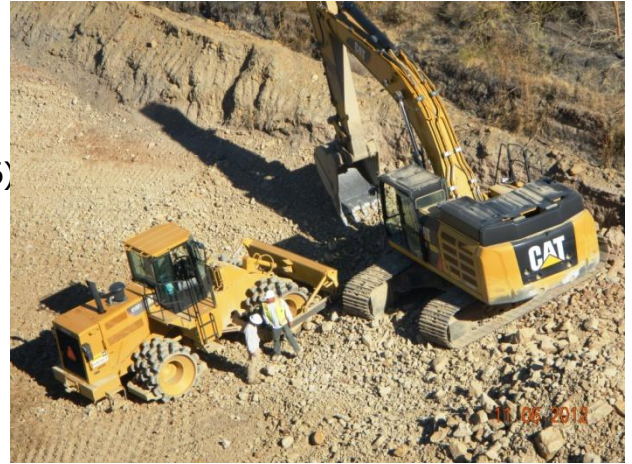
Subgrade preparation activities within the PBA Channel
