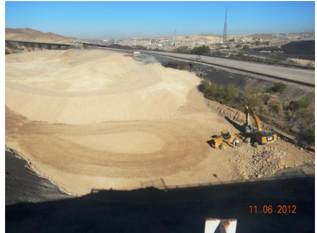
Existing conditions within PBA Channel
