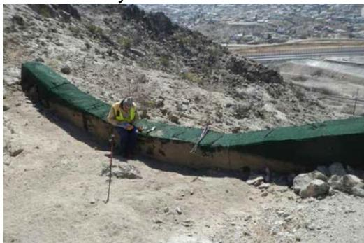
Photo 2 – Stormwater detained behind gabion
