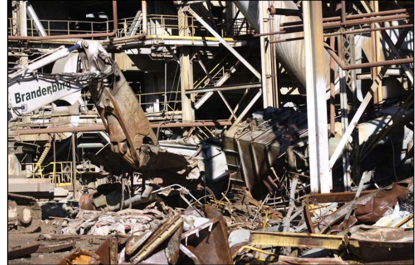
Dismantling of the reverberatory furnace.
