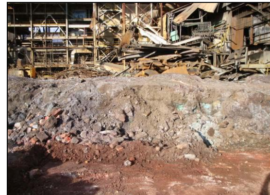
Copper matte exposed in the bottom of the furnace.
